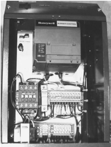
Figure 17. Control panel for the FDM burner on 1250-2400 (20:1 turndown) units
